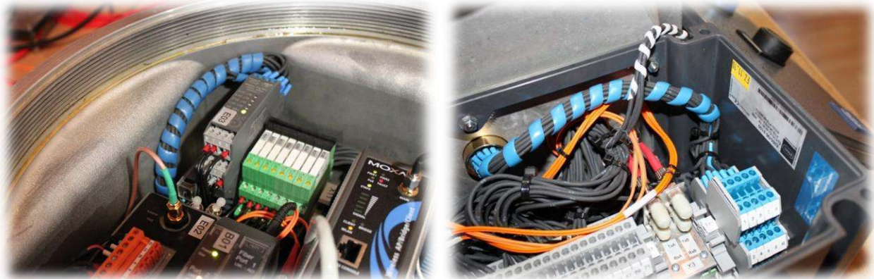
Fig.8.2: Intrinsically safe circuits of the ExConnection Rail
